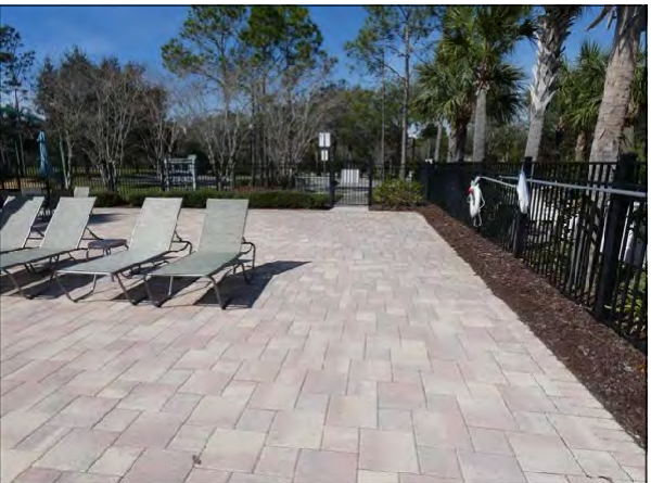
Pool Deck Pavers
