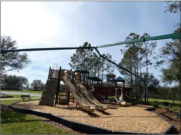
Tot Lot Shade, Missing From Recent Storm
